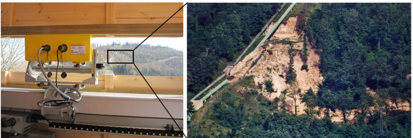
Fig. 4 Picture of the monitoring system (left) and picture of the landslide (right)
